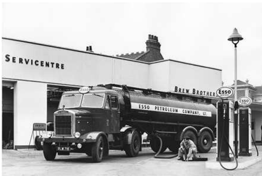
Figure 6: A Service Station in the 1950s (courtesy of ESSO)
